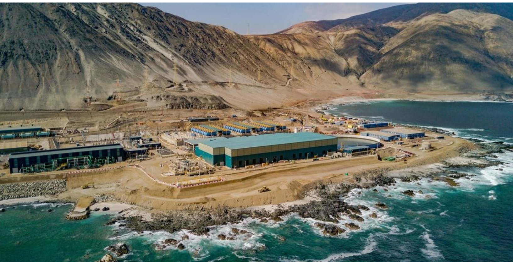
The 2,500lps desalination plant for Escondida in Chile
